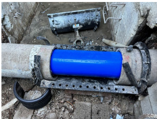
Figura 22 – Liner Primus Line in cameretta passante
